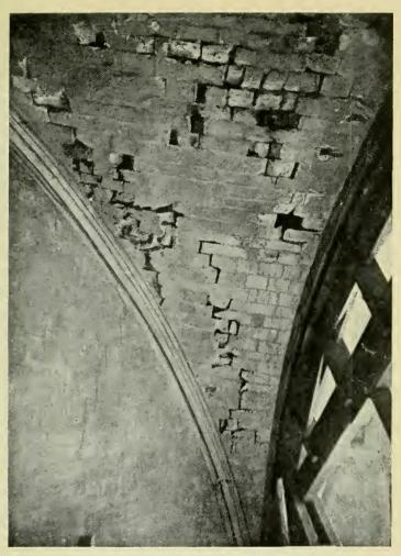
WINCHESTER CATHEDRAL. Showing the disintegrated condition of the masonry arches over the Presbytery.
